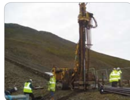
Keller – Wales Grout curtain creation at Marchlyn Mawr-Reservoir, Wales.
