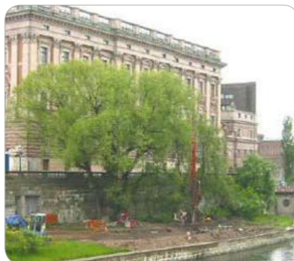
Parliament building, Stockholm – Sweden Construction of a 30 meter high grout curtain.
