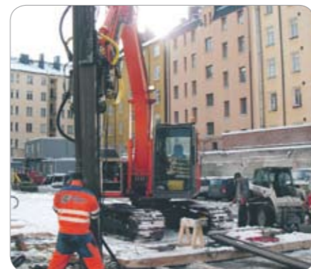
Munin, Stockholm – Sweden Foundation reinforcement work for a six-storey residential building.
